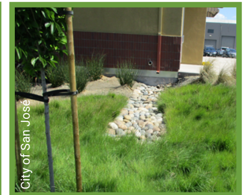
Well-placed cobble for flow dissipation
