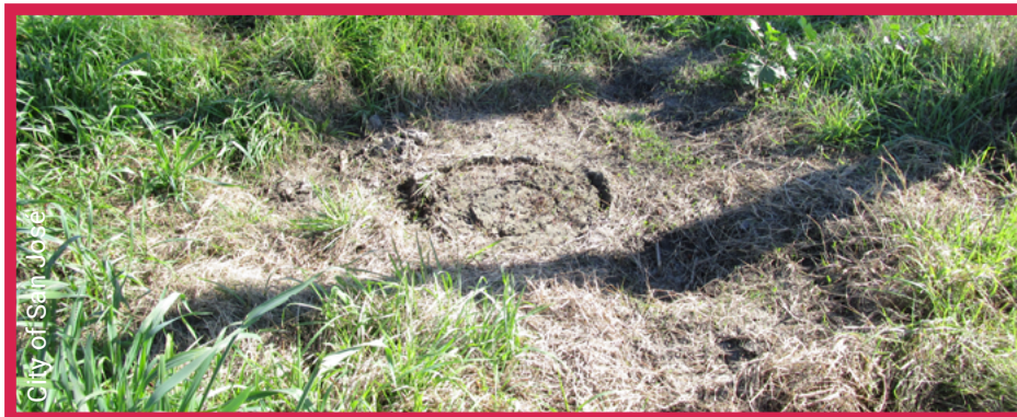
Vegetated GSI measure with significant deposited sediment
