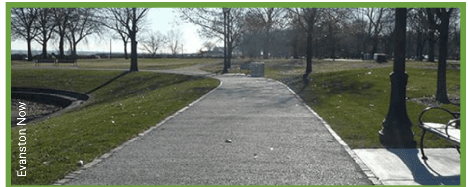
Pervious pavement with no structural damage
