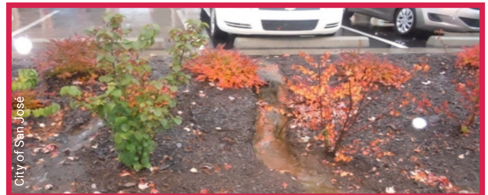
Evidence of erosion and channelization
