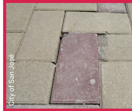
Interlocking paver with minor chipping
