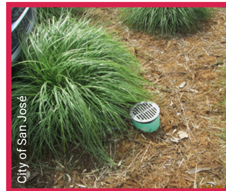
Inappropriate gorilla hair mulch
