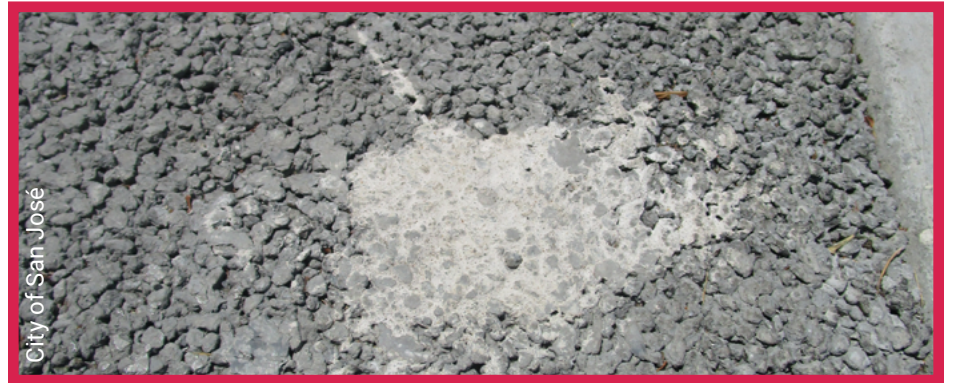
Pervious concrete with structural damage caused by concrete slurry
