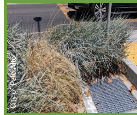
Cut back overcrowding of plants at overflow
