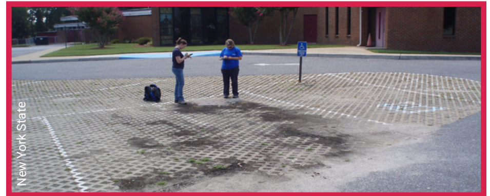
Pervious pavement in need of power washing
