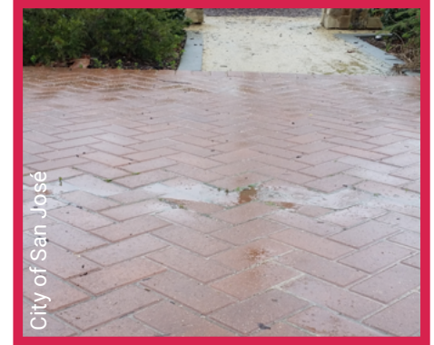
Pervious pavers showing signs of deterioration
