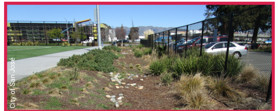
Vegetated GSI measure with poor plant density
