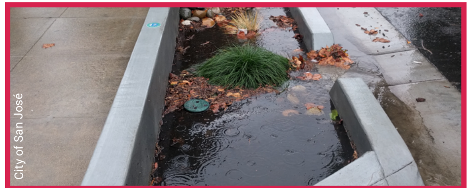
Leaf debris in curb inlet
