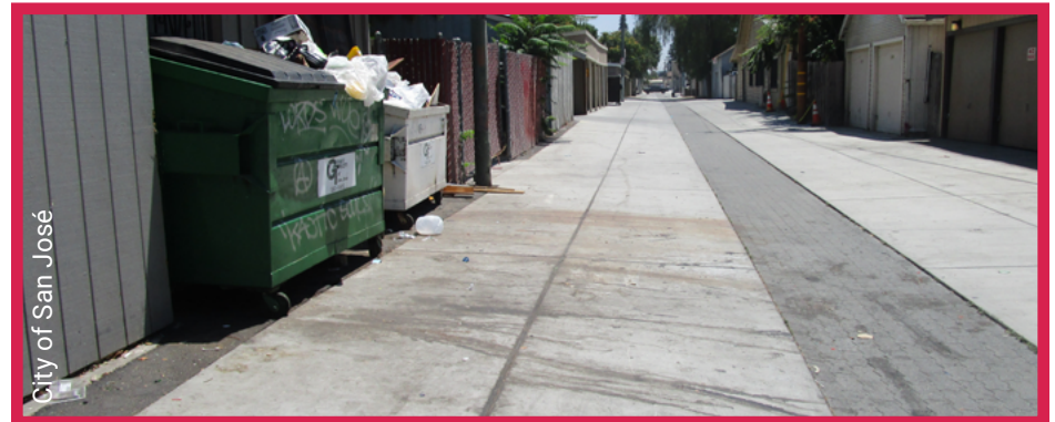
Dumpsters leaking leachate onto pervious pavement surface
