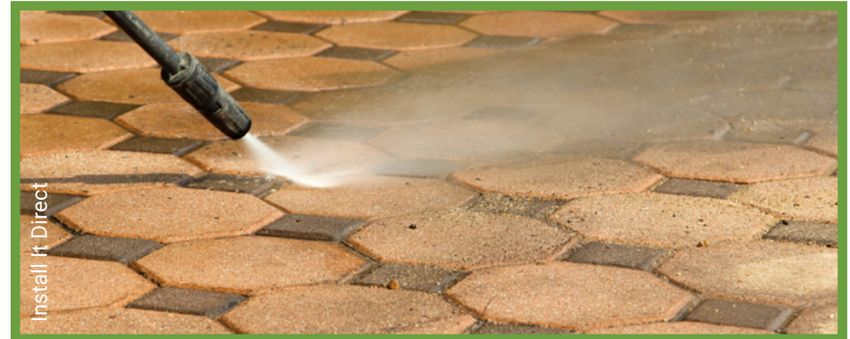
Power washing pervious pavement surface
