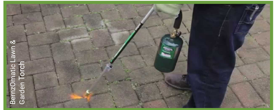
Weed burner to restore pervious pavement surface performance
