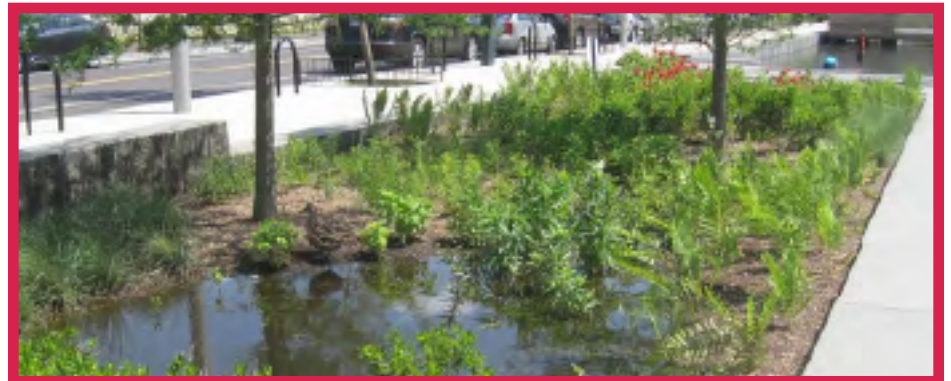
Bioretention planter with standing water 24 hours after rainfall
