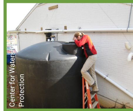
Inspect and note sediment accumulation
