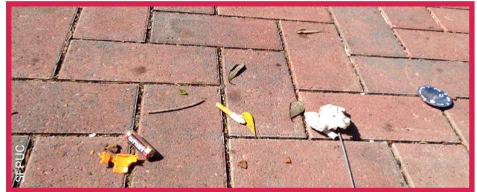
Trash and debris on pervious pavement surface
