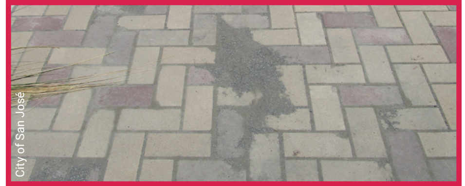
Pervious pavement surface clogged with sediment
