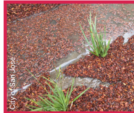
Bark mulch floating into overflow of treatment area
