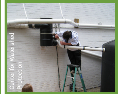
Inspect piping and valves
