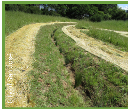
Erosion control Best Management Practices installed adjacent to a vegetated GSI measure
