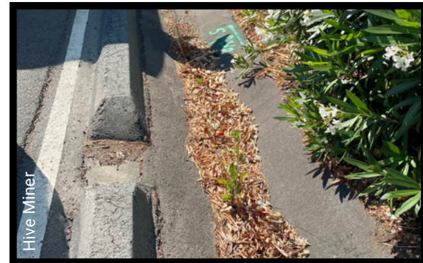
Well-maintained infiltration trench
