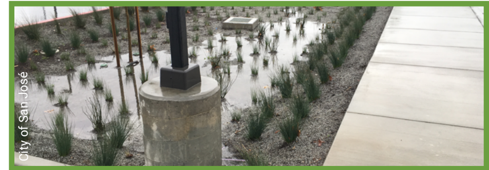
Vegetated GSI measure with minimal standing water and optimal infiltration
