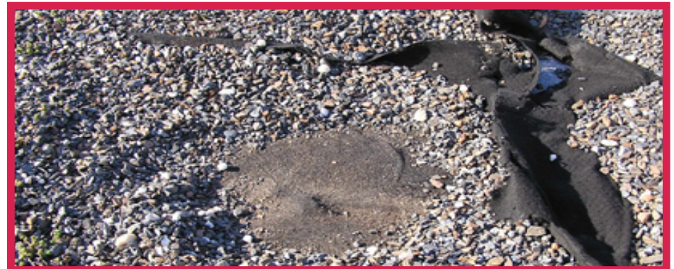
Do not allow damaged membranes to go unrepaired
