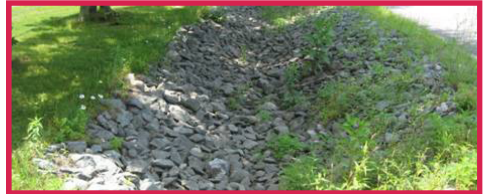
Unkempt cobble infiltration trench
