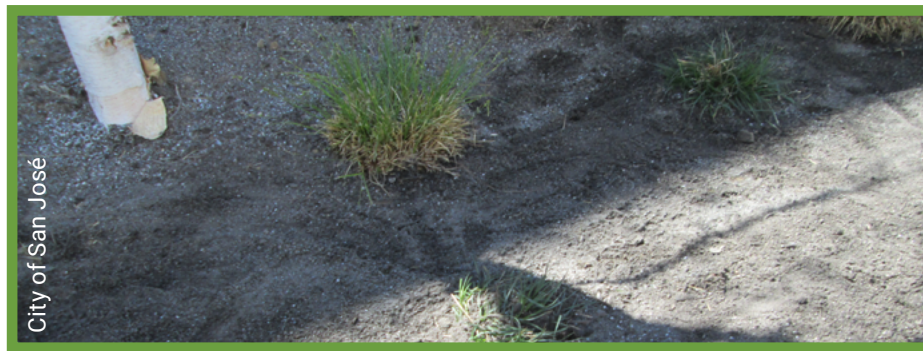
Sediment manually removed from vegetated measure
