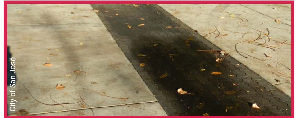
Clogged pavers with ponding
