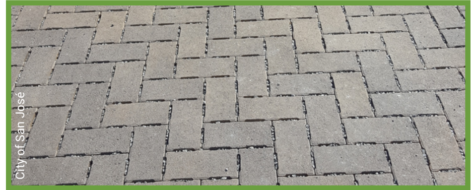
Newly installed pervious interlocking concrete pavers
