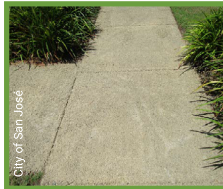
Cleaned pervious concrete sidewalk
