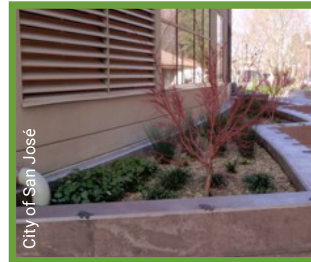
Properly planted flow-through planter
