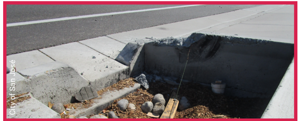
Curb damaged by heavy equipment
