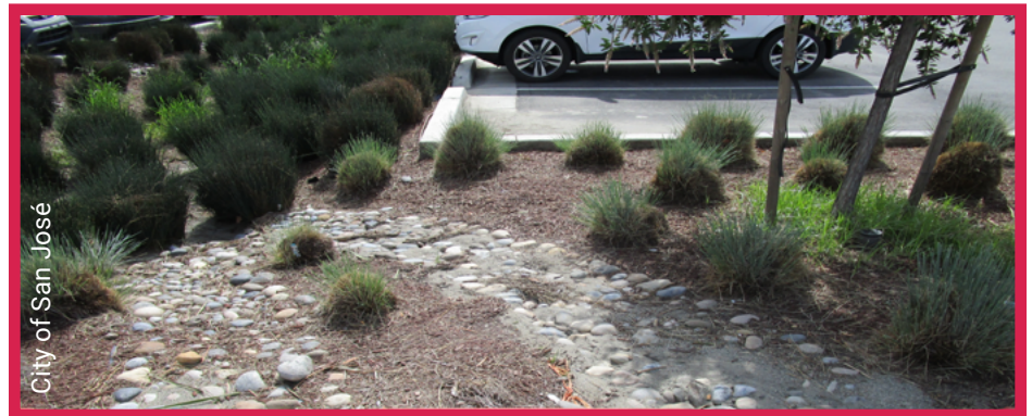
Cobble severely impacted by sediment
