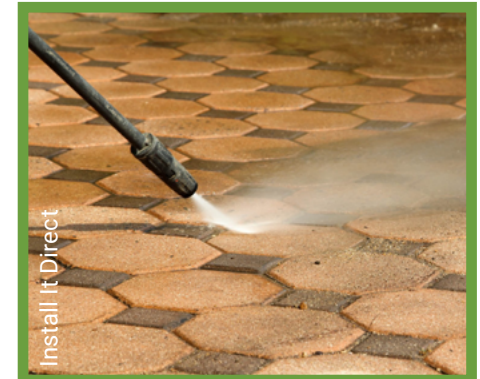
Power wash pervious pavement surface
