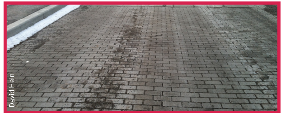
Pervious pavement in need of vacuuming
