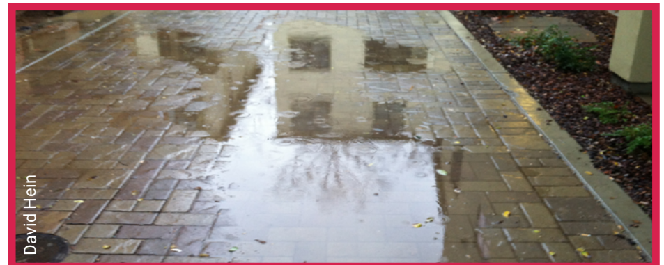
Pervious pavement with standing water
