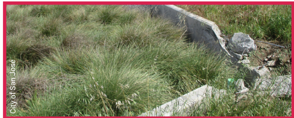
Treatment area damaged by vehicular traffic
