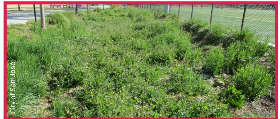
Bioretention area with significant weeds
