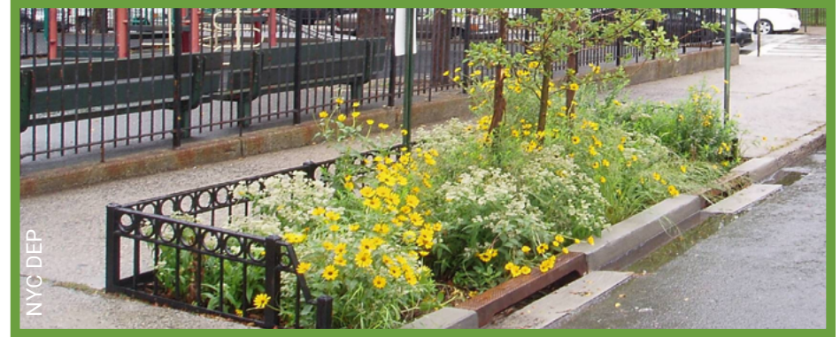
Treatment area with structural barrier in good condition
