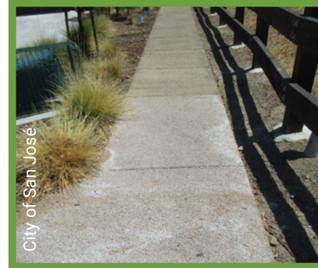
Installed pervious concrete sidewalk
