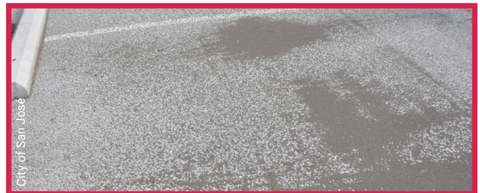
Pervious pavement with sedimentation blocking drainage
