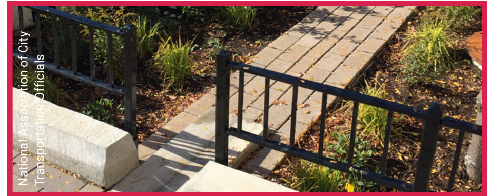
Gap in fencing that promotes pedestrian accesses through bioretention area
