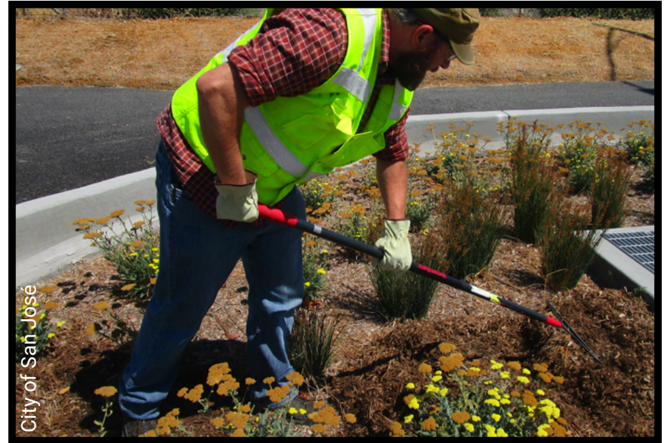
Spreading mulch in bioretention planter with proper tools
