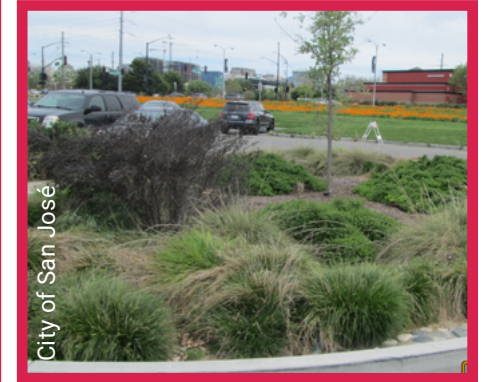
Dead ceanothus in a bioretention area
