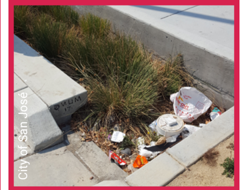
Significant trash in vegetated GSI
