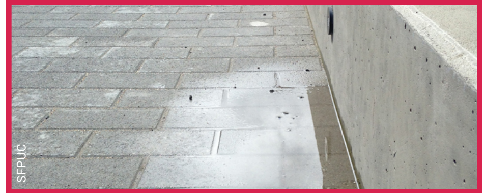
Clogged pavers with ponding
