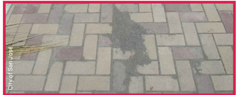
Pervious pavement surface clogged with sediment
