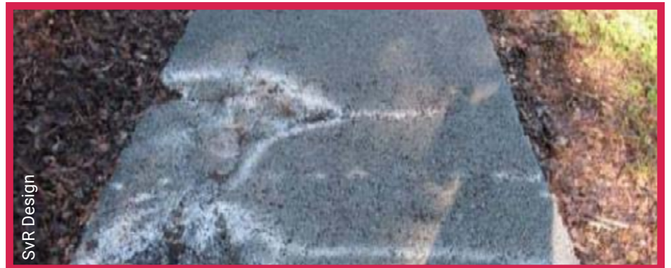
Pervious pavement sidewalk with structural damage
