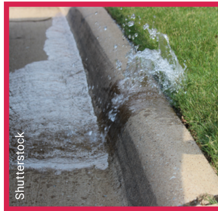
Damaged sprinkler head
