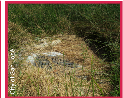
Overgrown grasses blocking overflow
