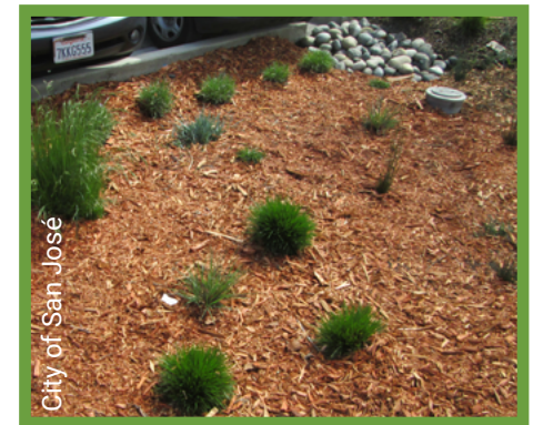
Install 3" of fresh arbor mulch with plantings
