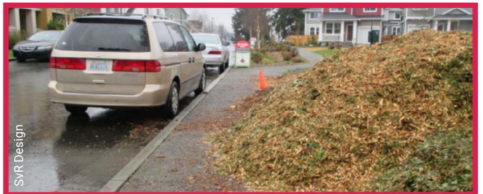
Pervious pavement with landscape debris stockpiled on surface
