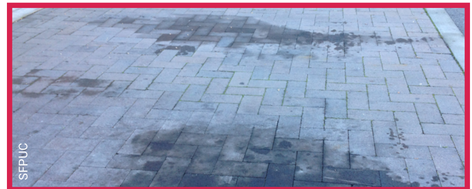
Pervious Pavement with oil staining
