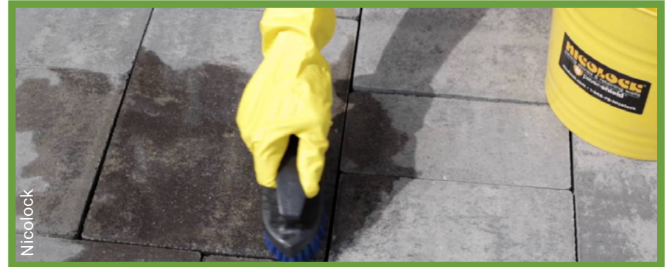
Removing oil from permeable brick pavers
