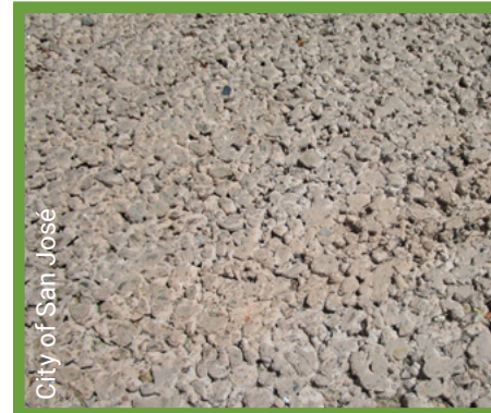
Pervious concrete free of sediment
