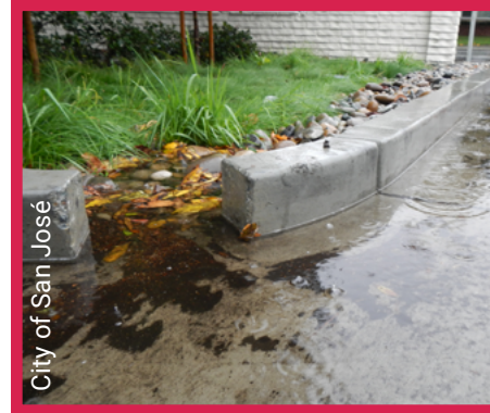
Leaf debris blocking curb inlet
