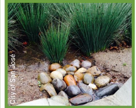
Clean and well placed cobble at a curb inlet
