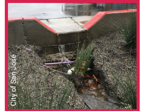
Severe erosion at the inlet of bioretention area
