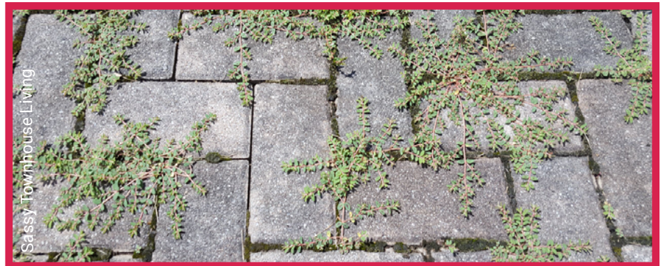
Pervious pavement with nuisance plant growth
