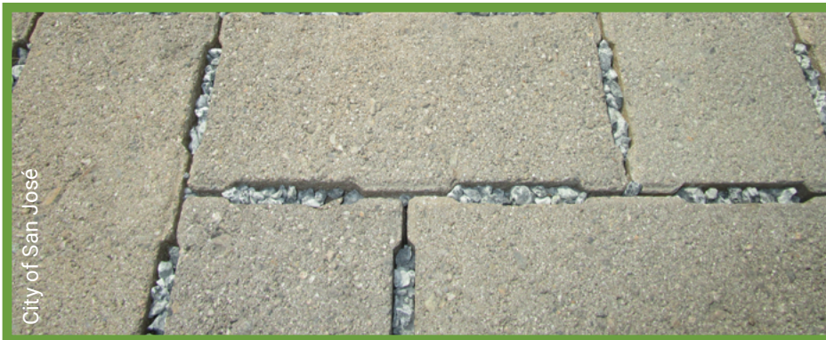
Pervious pavement with no sedimentation
