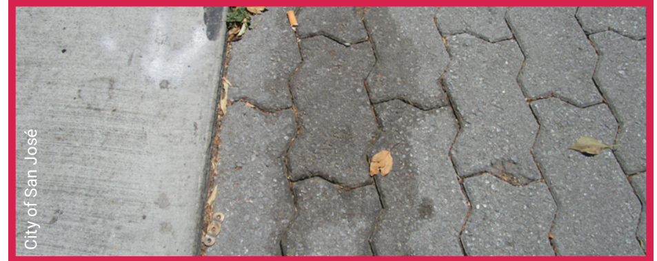
Contaminant staining on Pervious Pavement surface
