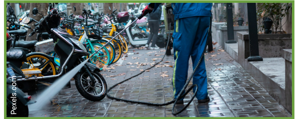
Pressure washing pervious pavement surface
