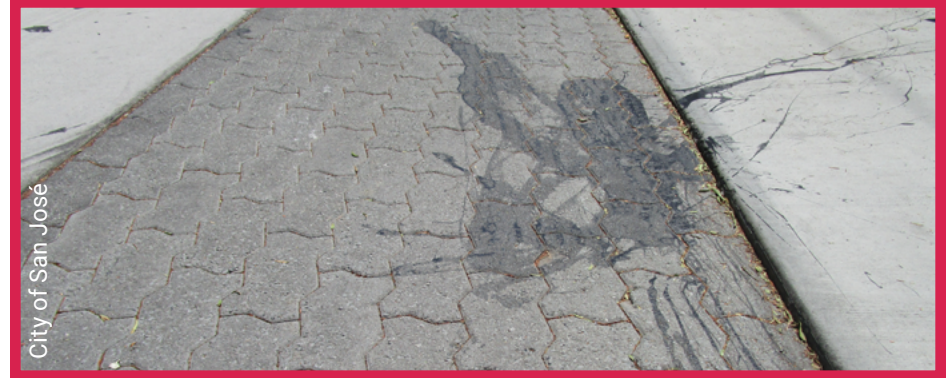
Contaminants dumped on pervious pavement surface
