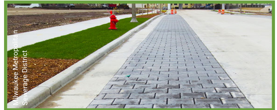
Pervious pavement with no standing water
