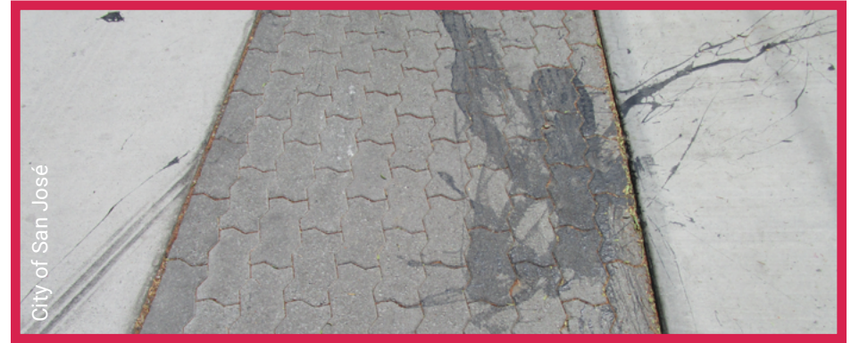
Paint staining on Pervious Pavement surface
