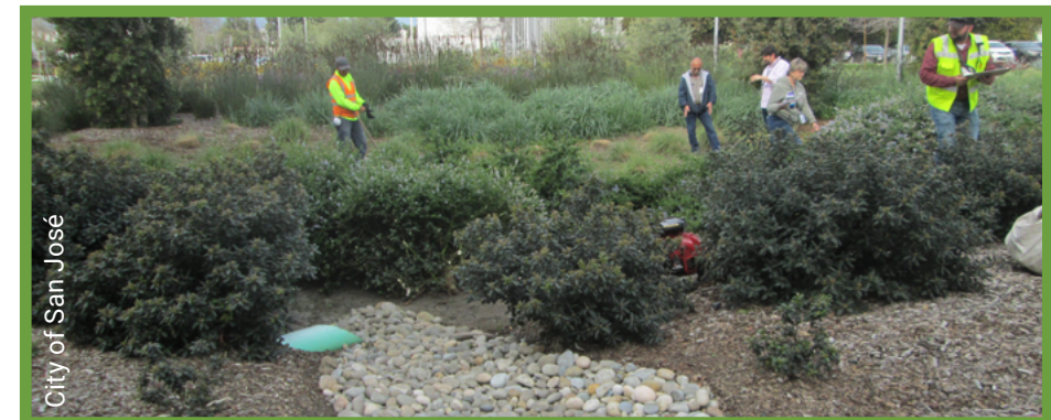
Vegetated GSI measure with adequate and clean cobble at inlets
