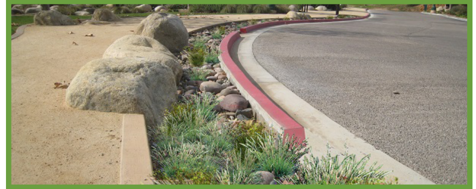
Properly maintained infiltration trench
