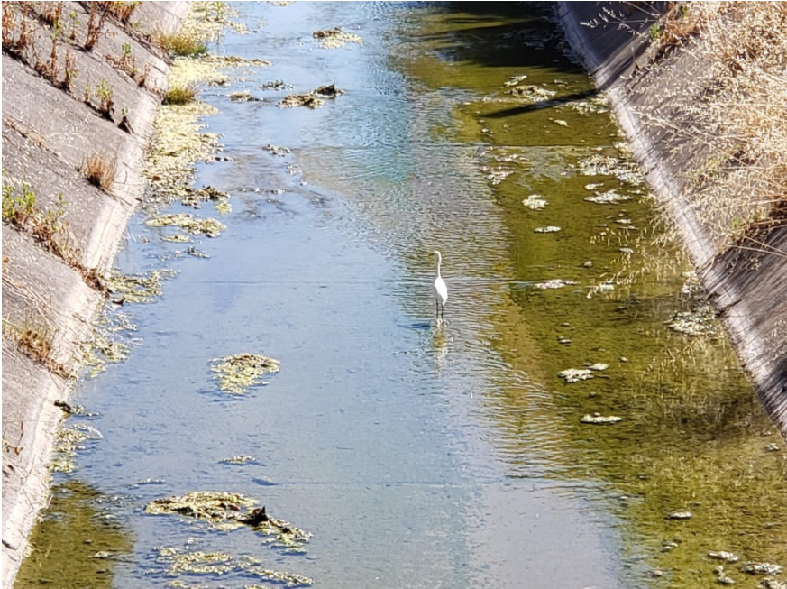
Matadero Creek at Ross looking upstream:
