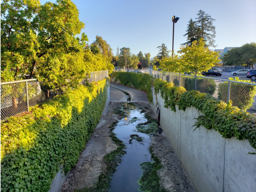
Matadero Creek at Park Ave looking upstream:
