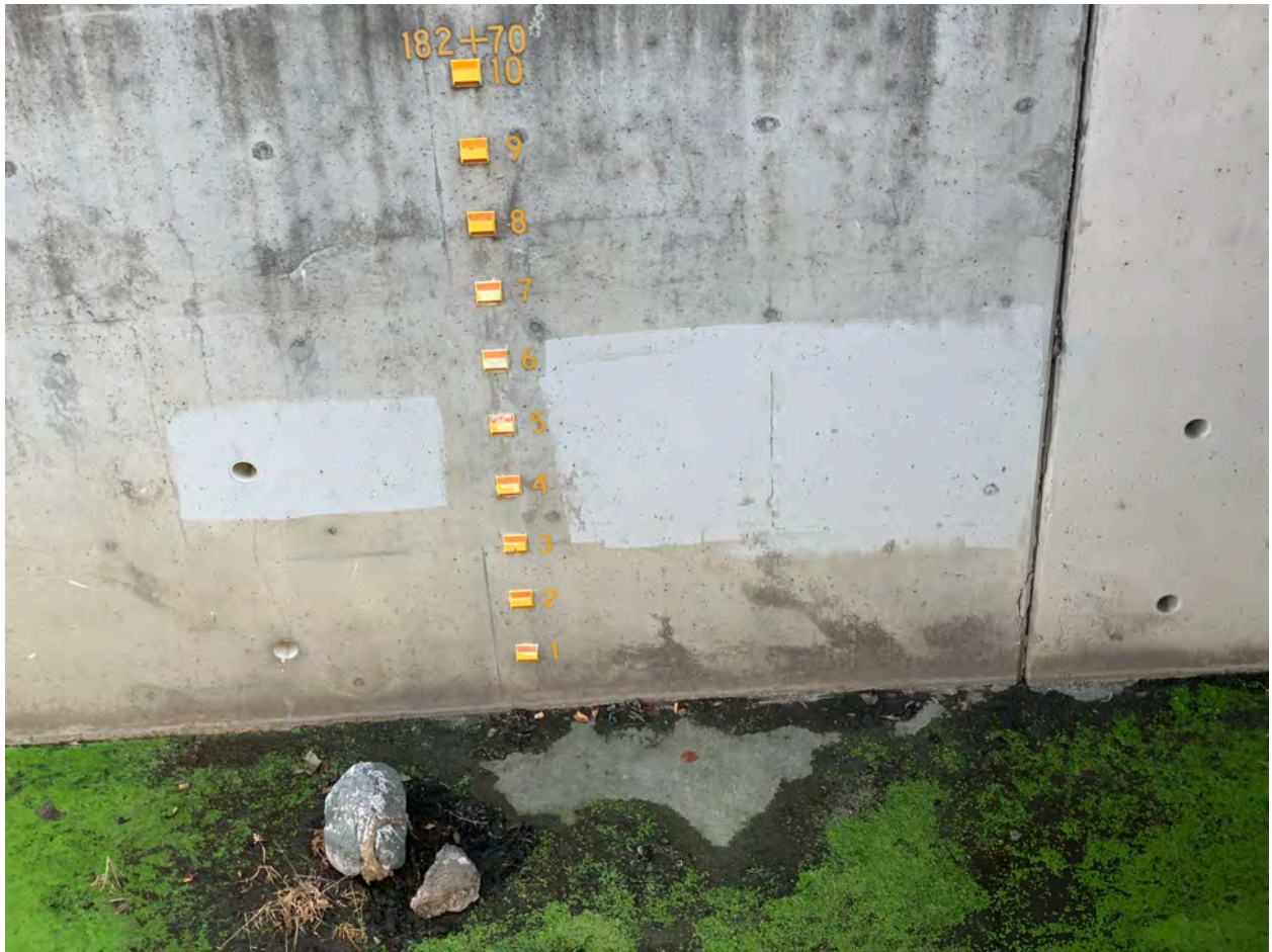
Figure 7 Channel Station and Water Surface Elevation with low flow conditions
