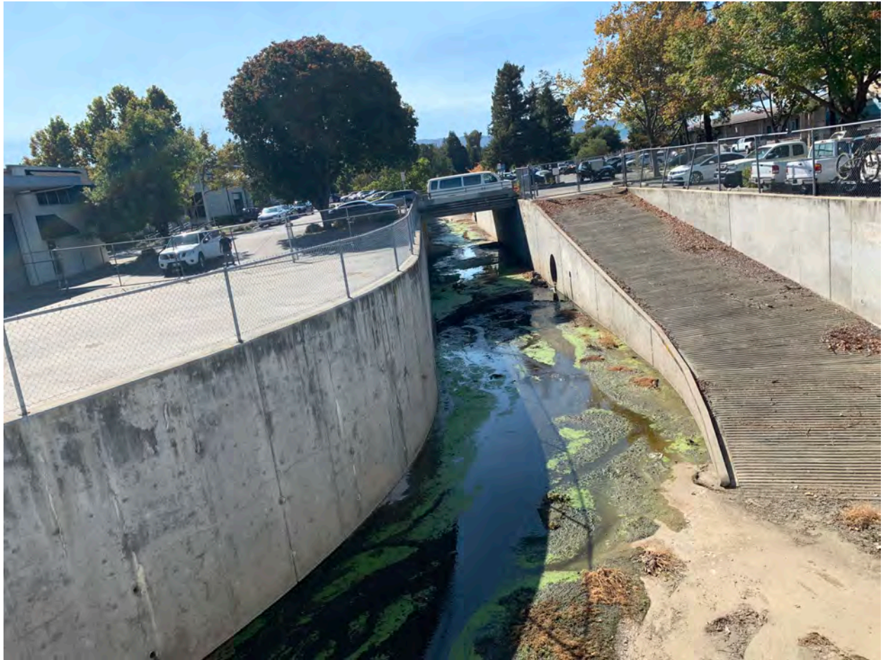
Figure 12 Concrete Channel under Lambert Boulevard Bridge with Existing Valley Water Maintenance Access from street
