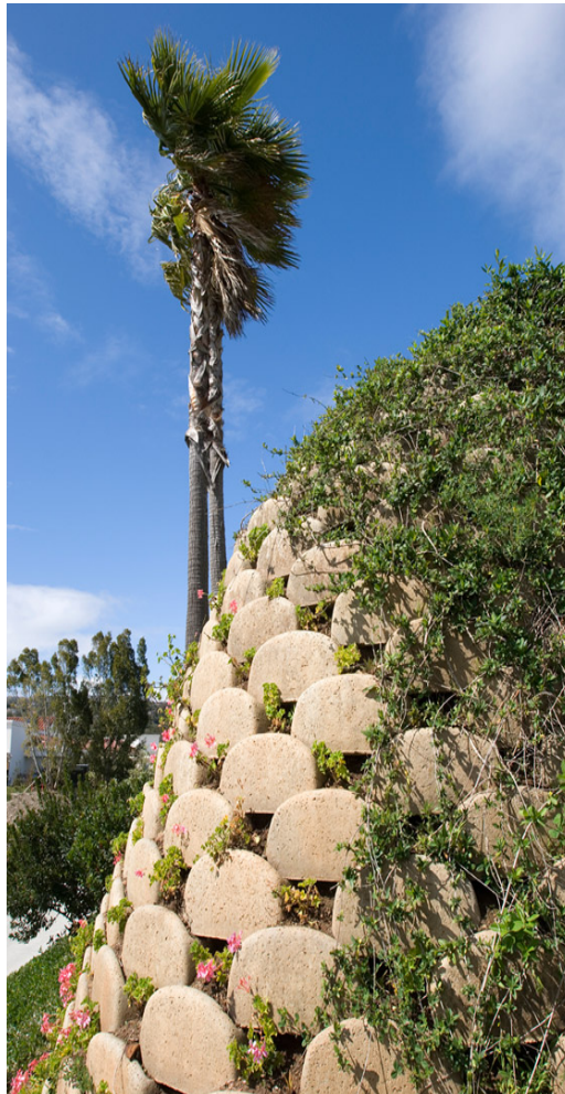
Figure 8. Example of plantable concrete retaining wall structure in San Diego, California (Soil Retention, 2020)
