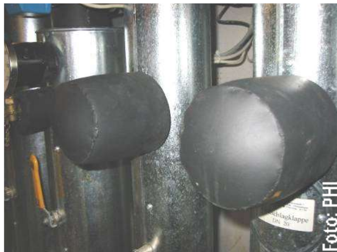
Fittings covered by insulating mouldings. Prefabricated insulating mouldings are available by now.
