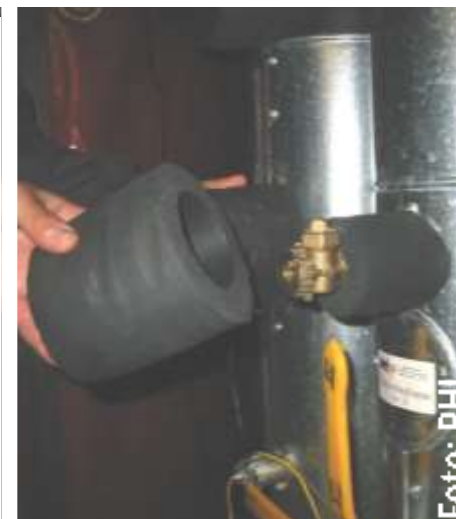
Fittings covered by insulating mouldings. Prefabricated insulating mouldings are available by now.
