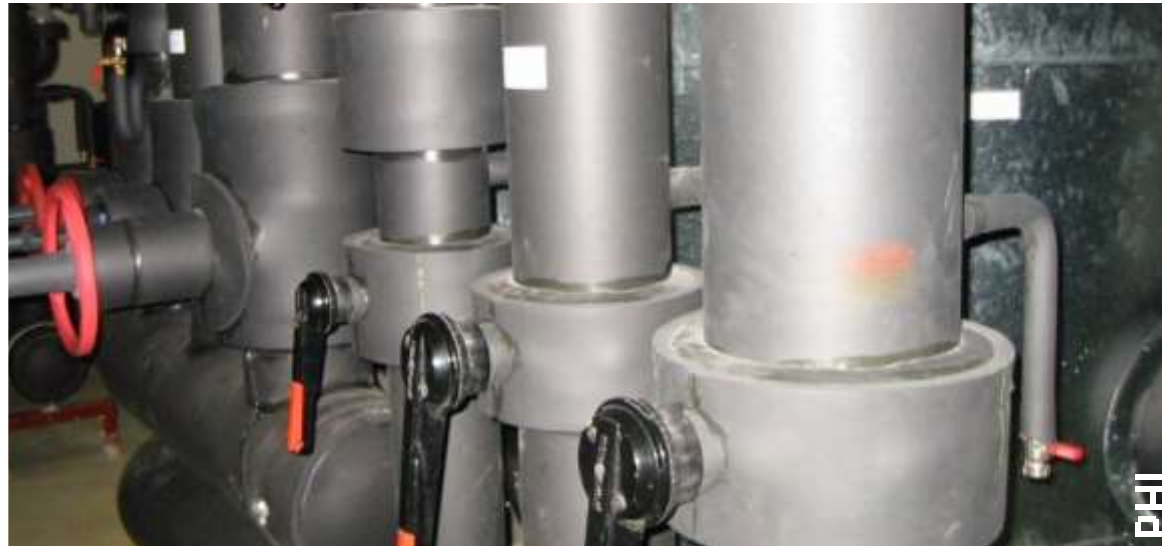
Fittings covered by insulating mouldings. Prefabricated insulating mouldings are available by now.
