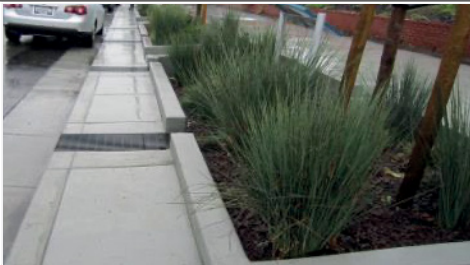
Bioretention with vertical walls located in parkway with step out zone for passengers exiting parked cars in El Cerrito (SFEI, 2012)
