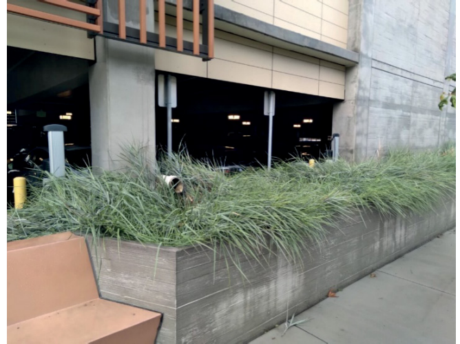
California Avenue Parking Garage Flow-Through Planter, City of Palo Alto
