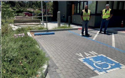
Parking Stall Pavers at Fire Station #3, City of Palo Alto
