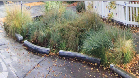
Bioretention bulb-out at Kellogg and Middlefield, City of Palo Alto
