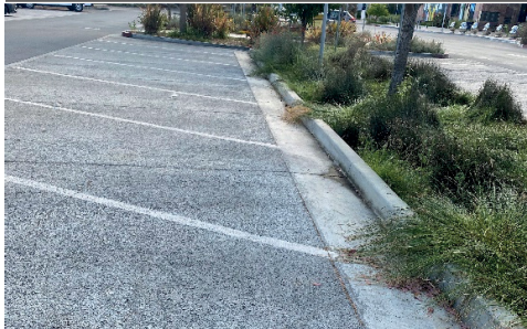
Porous Concrete at Mitchell Library Parking Lot, City of Palo Alto
