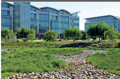
Example of Regional Treatment Facility when Dry at Pacific Shores Center in Redwood City, California (DES Architects +Engineers)
