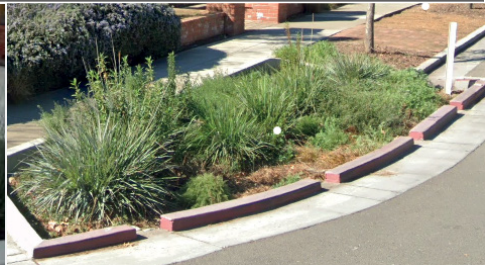
Bioretention bulb-out in Southgate neighborhood with parking not allowed, City of Palo Alto
