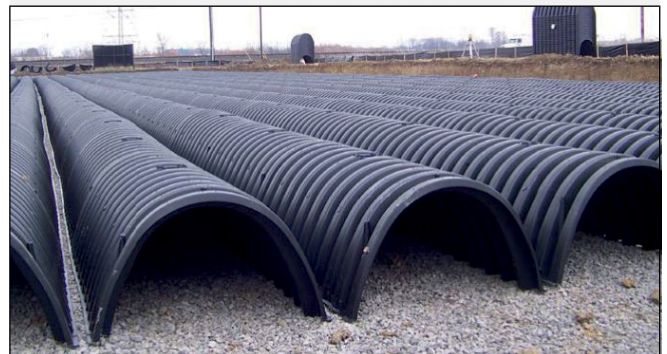
Example of a subsurface retention/ infiltration system installation under a parking lot (Conteches.com)
