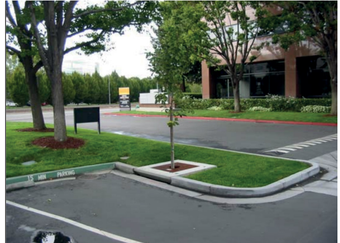
Tree well filter, City of San Jose (SCVURPPP C.3 Guidance, 2024).
