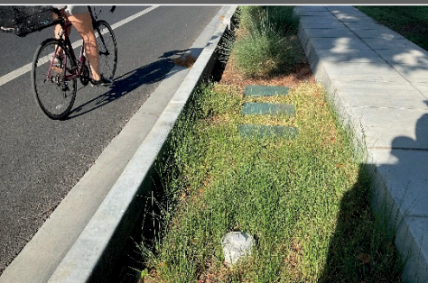
Bioretention adjacent to bike lane located at Charleston-Arastradero, City of Palo Alto
