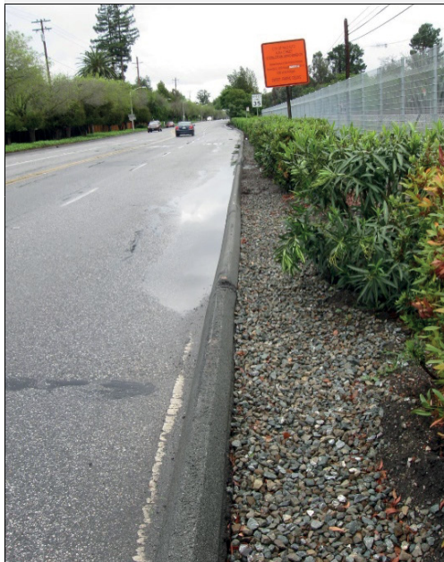
Example of an infiltration trench, Alma Street, City of Palo Alto
