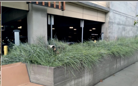
Flow-through Planter adjacent to California Avenue Parking Structure, City of Palo Alto
