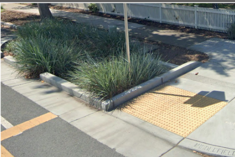
Bioretention bulb-out integrated with ADA curb ramp crossing at Kellogg and Middlefield, City of Palo Alto
